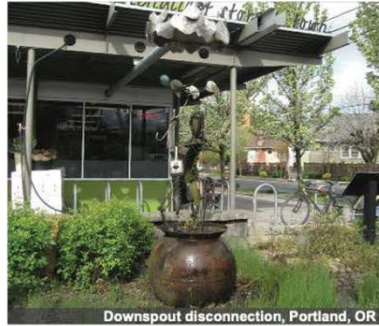
Downspout disconnection, Portland, OR
